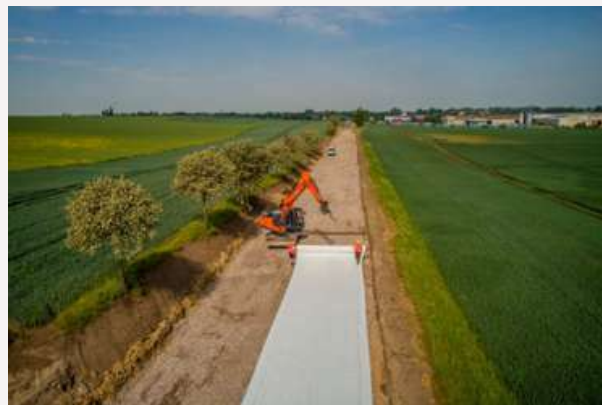
Figure 2: Use of geosynthetics to stabilize embankments over peat/swamp soils, mitigating settlement and improving stability
